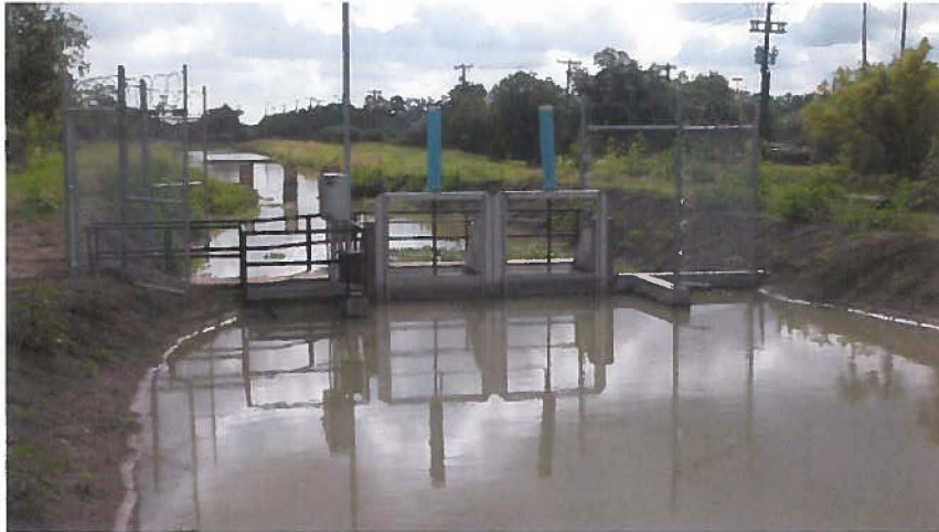
Picture 1. Dual gate canal check at the diversion to the municipal water supply.
